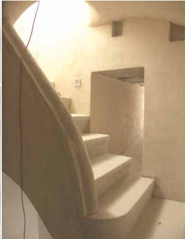
Fig. 60 View of the Bell Tower after the 2003/06 restoration works.
