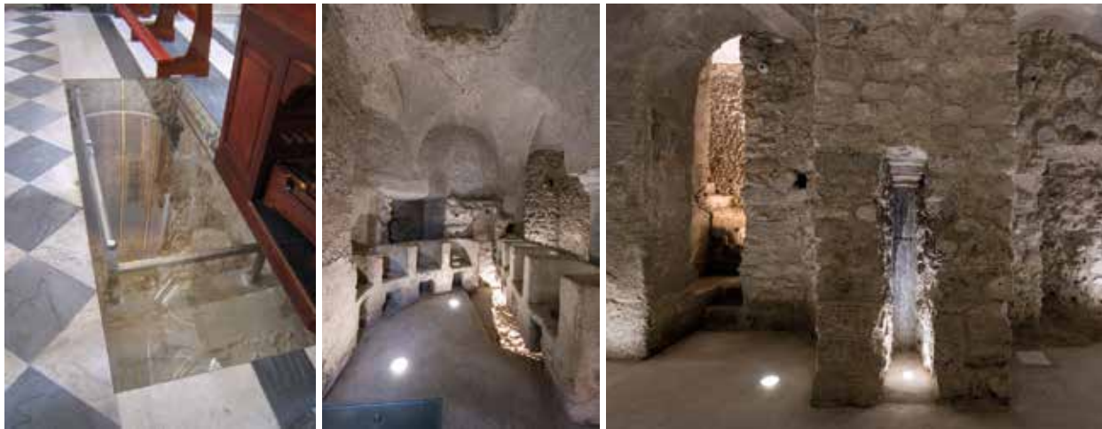
Fig.42 Current floor closing hatch of the staircase leading to the lower crypt from Chiesa di Santa Maria Assunta. It is made of tempered glass and a stainless steel structure and characterised by a lime screed with colourful mosaic tesserae and it is completely independent from the perimeter masonry.
