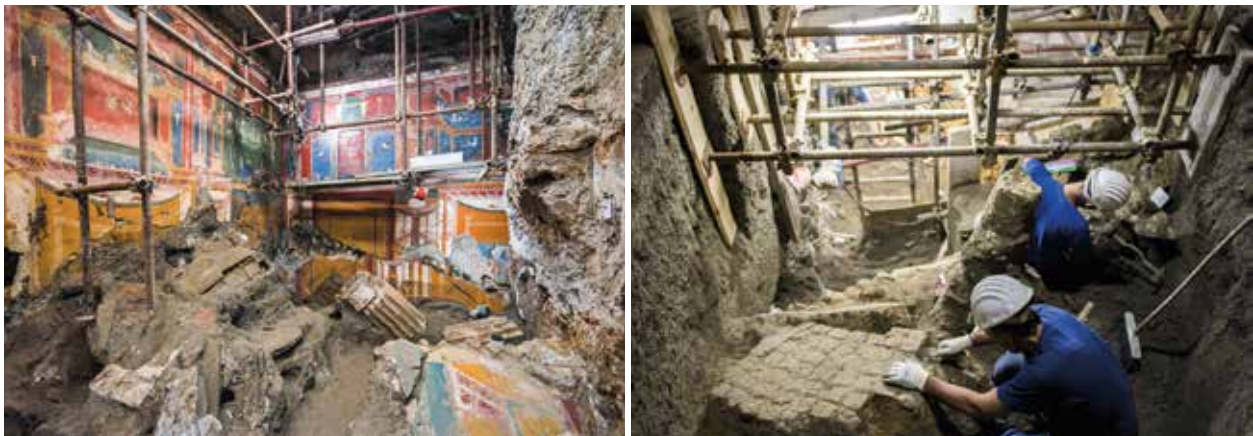
Fig. 3 Emergency interventions made by the restorers during the archaeological excavation
