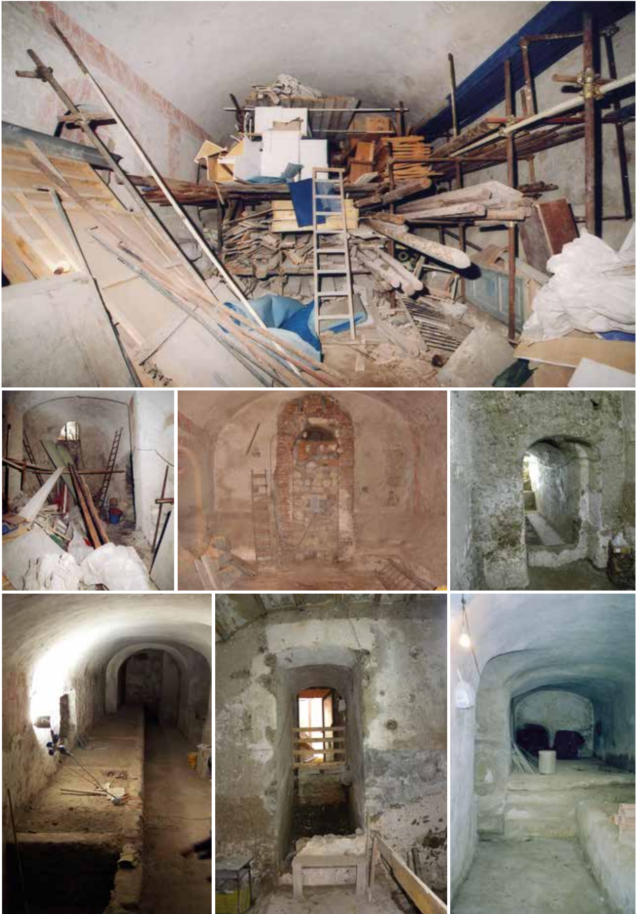
Figs. 6-12 Photos of the upper Crypt before the 2003/06 works. You can see the room conditions after the removal of the building materials showing the walled up passage to Piazza F. Gioia used as division from the Enel room still working till May 2006.
