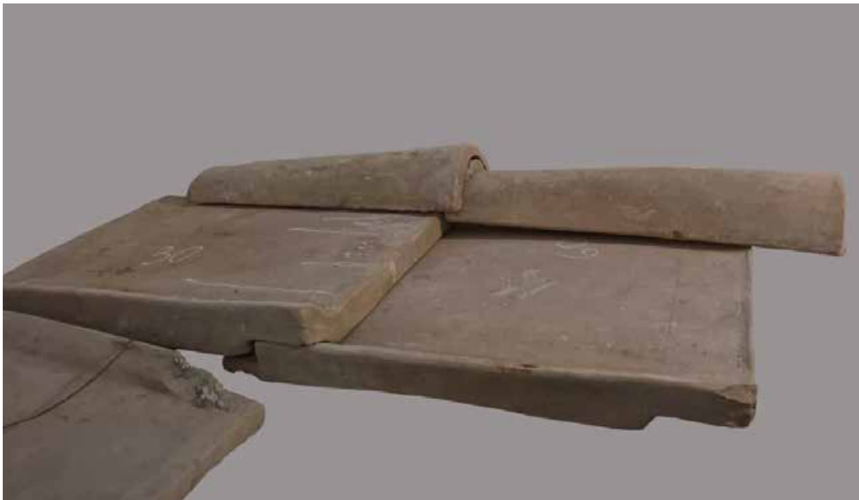
Fig. 20 Detail of the roof original recess clay-bricks of the 1 st cent. BC Roman villa.
